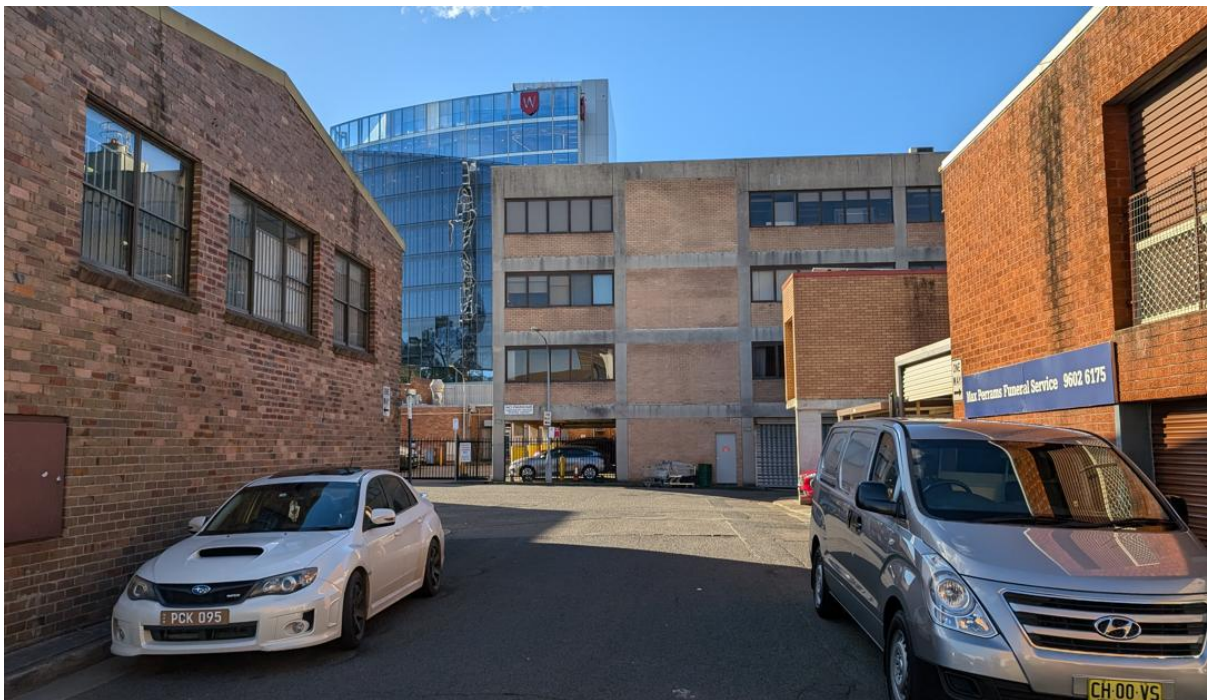
Figure 14: View toward the rear of the Elizabeth Street portion of the site from Hanwell Serviceway
