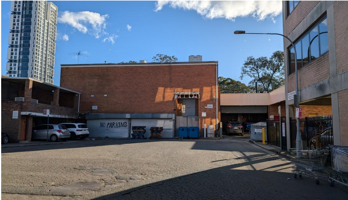
Figure 13: View from Hanwell Serviceway toward the rear of the Macquarie Street portion of the site and part of the area associated with the land swap
