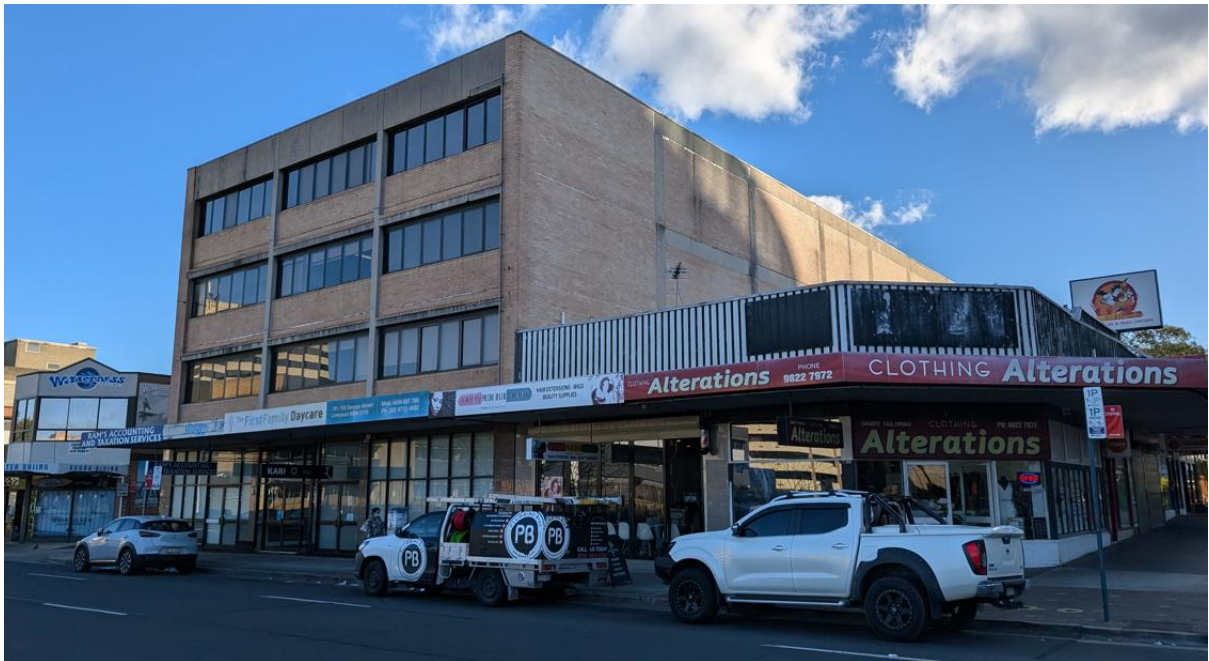
Figure 6: View of the George Street portion of the site
